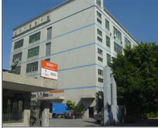
External photo(s) of the production unit(s) factory gate and production building.JPG
