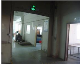
Photo of fire safety equipment safety exit.JPG
