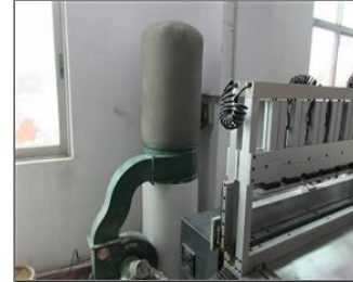
Photo of the inside of the main production hall Dust collector.JPG
