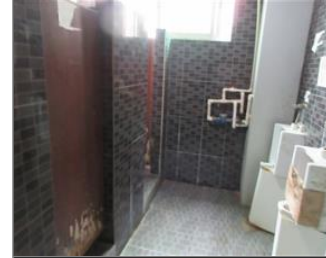
Photo of the sanitary facilities Toilet.JPG
