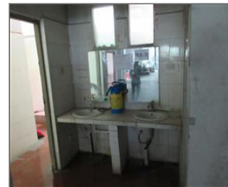
Photo of the sanitary facilities Hand wash station.JPG
